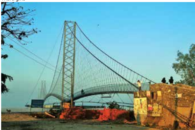
Mahakali suspension bridge
